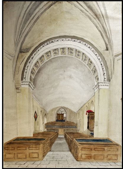
St Mary's looking west from the chancel showing the forward facing pews and the pulpit, The plaster was later stripped from the walls and ceiling
