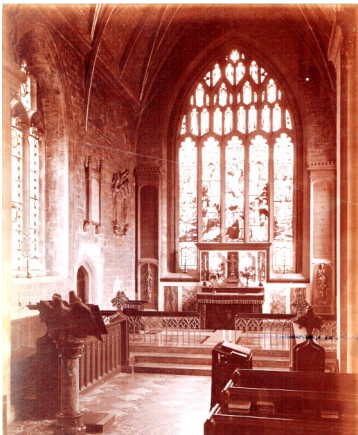
This photograph was taken in the early twentieth century and shows that the choir stalls were then located in the Chancel at the front of the church
